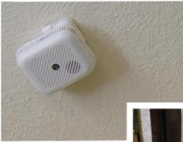
Smoke and CO alarms can be added to any system to alert the Carer to an emergency. Ionisation and optical smoke alarms are available.
